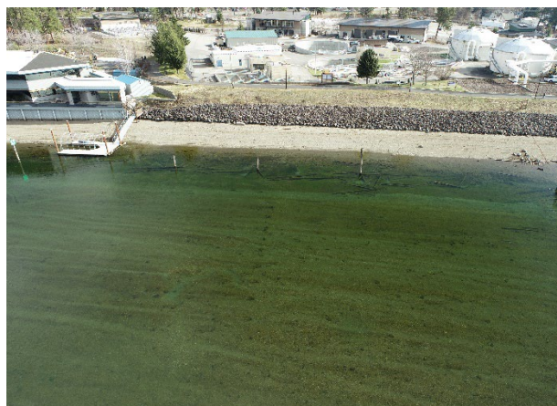
Spokane River, Coeur d'Alene, Idaho. City of Coeur d'Alene Advanced Wastewater Treatment Plant Effluent Diffuser Ports.
