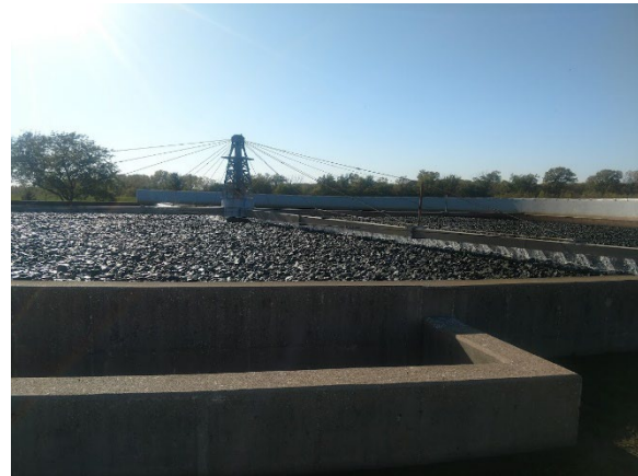
Rock Media Trickling Filter.
