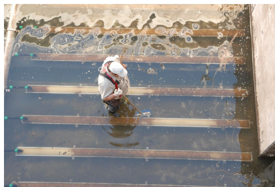
Improve Efficiency with New/Clean Diffusers. Reprinted with permission from Michael Stenstrom.
