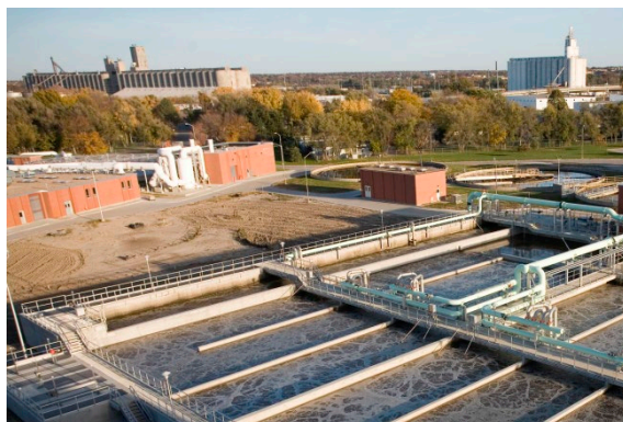
Pre-nitrification Zone (top zone) with Return RAS and to Nitrify Reject Water to BNR Basin.
