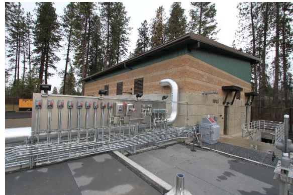
Tertiary MBR with Chemical P Removal to Low Levels.
