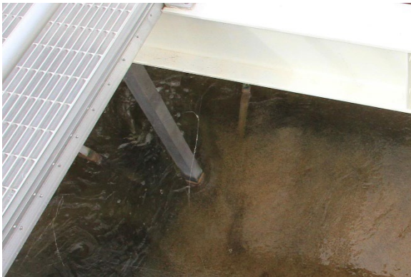
Actiflo for Tertiary P Removal.
