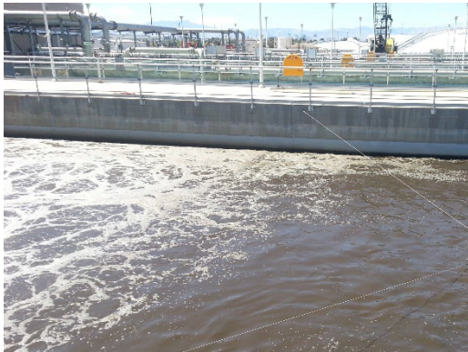
Dissolved Oxygen Carryover from Aerated to Unaerated Zone.
