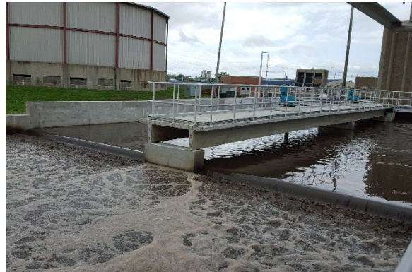
Aeration Tanks Converted to BNR
